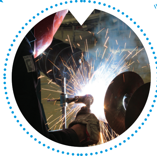
Applying Wear Protection
